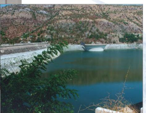
Average water discharge Average production Dam height Installed capacity 30.40 m3/s 220 GWh 105 m 116 MW
